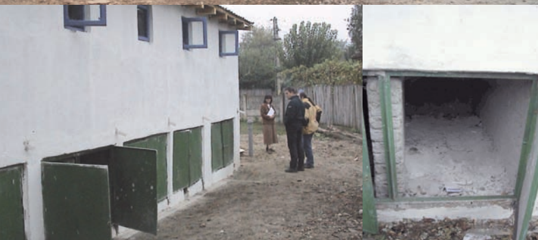
View on the new toilet facility from the back with open doors to the double vault faeces chamber
