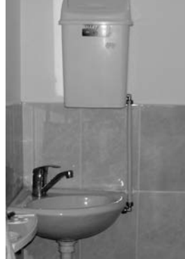
Example of handwash basin without central water supply from Moldova
