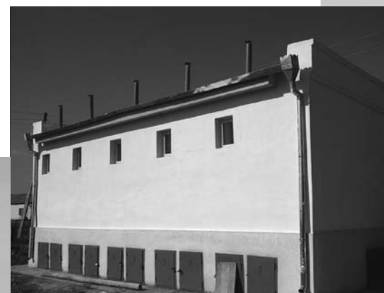
UDD toilet facility with passive ventilation
