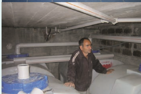
The caretaker in the basement where four urine tanks (each 2 m 3 ) are installed (photo by AWHHE)
