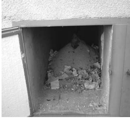
Well maintained double-vault faeces collection with insulated door
