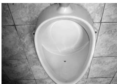
Conventional urinal is used as a waterless one, the holes were sealed apart from one left
