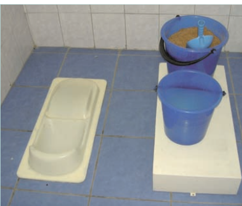
View into a restroom with the installation of the Chinese squatting slab
