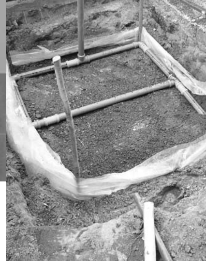
Greywater treatment in simplified filter
