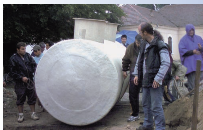
Installation of the double chamber urine tank (made of glass-fiber laminate) into the ground
