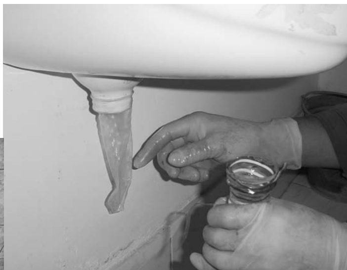
Installation of a smell trap in the urine pipe under the waterless urinal
