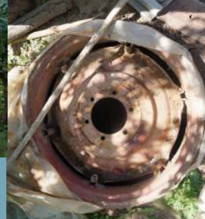
Soak pit installed by a villager in his yard for the treatment of the wastewater (An-Oston village)
