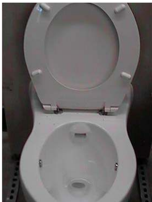
Vacuum toilet using one liter per flush
