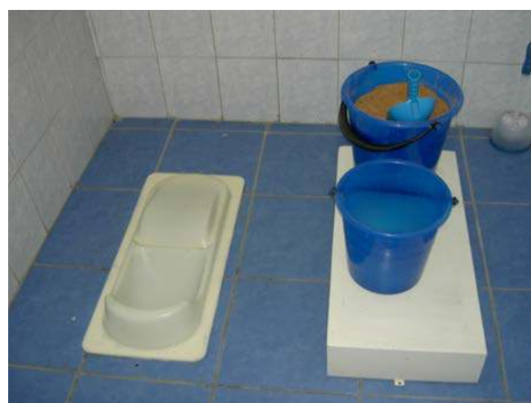
Interior of a UDDT cabin
