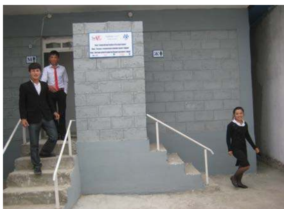
Separated toilet facilities for boys and girls
