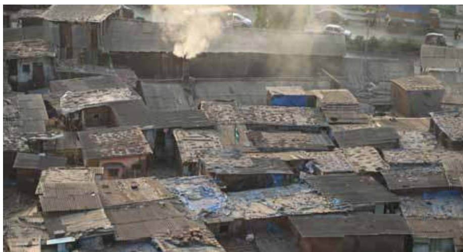
Asbestos containing roofing materials, © ROCA/GAAA
