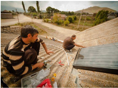
Photos: Building and installing solar collectors in Armenia (copyright: Beyond Borders Media) and Belarus
