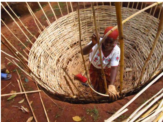
Photo: Women's traditional skills are required in building the framework for the dome of the biogas plant
