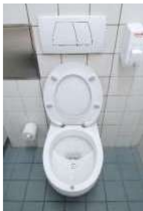
Urine diverting toilet with water flush (source: Pixabay)
