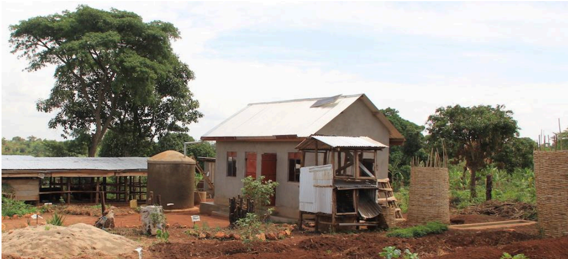
ARUWE's demonstration farm with bio- and water tanks made out of bamboo.
